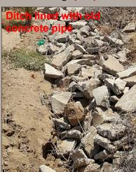
The roadside gully formed because the water velocity increased as the hill steepened. Gravel in the existing gully will protect the gully from eroding further. Riprap at the start of the downslope will help to dissipate excess energy as water begins to flow downhill.
